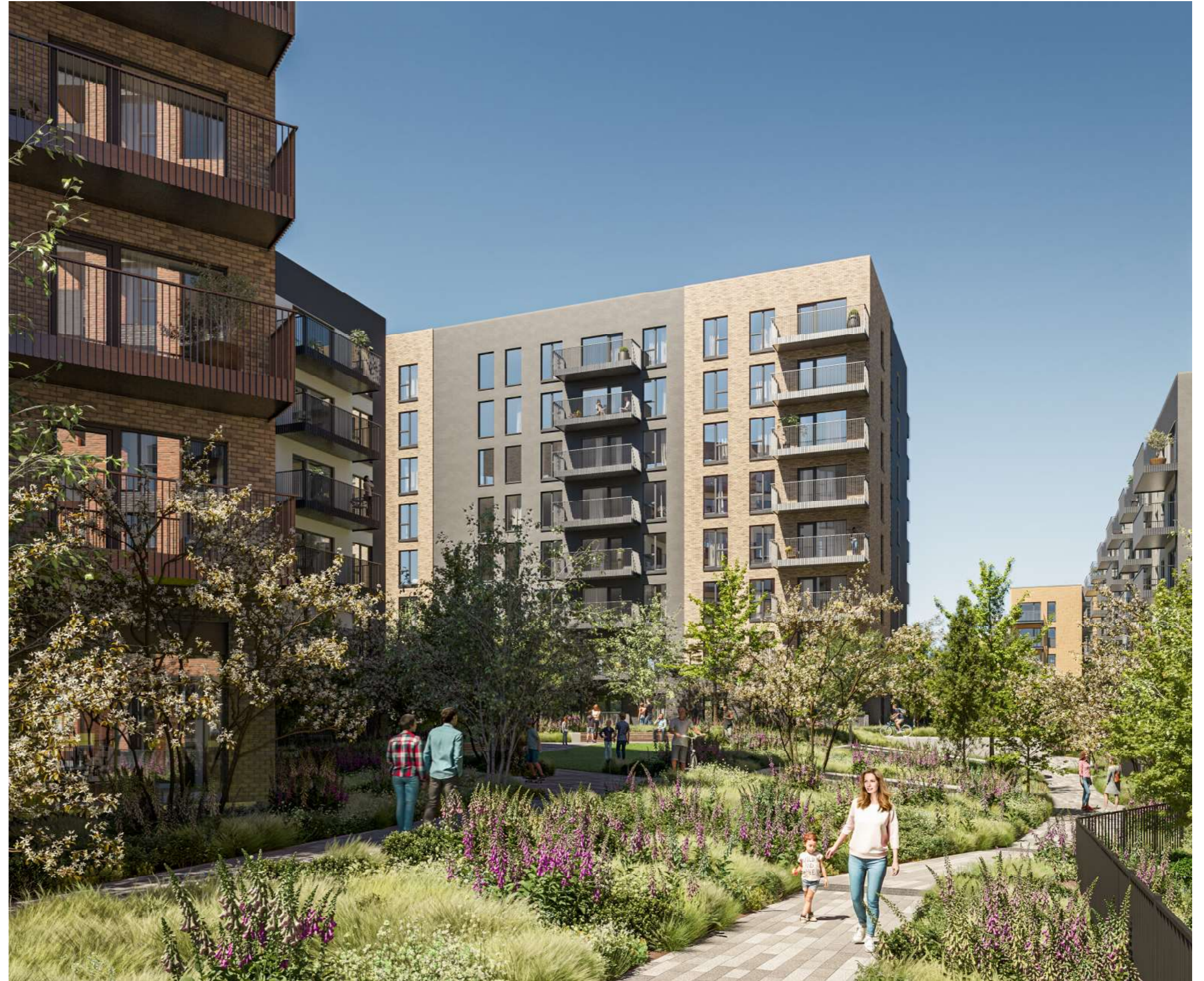
Figure 3 - View of western communal open space between Blocks D4, D3 and D2
