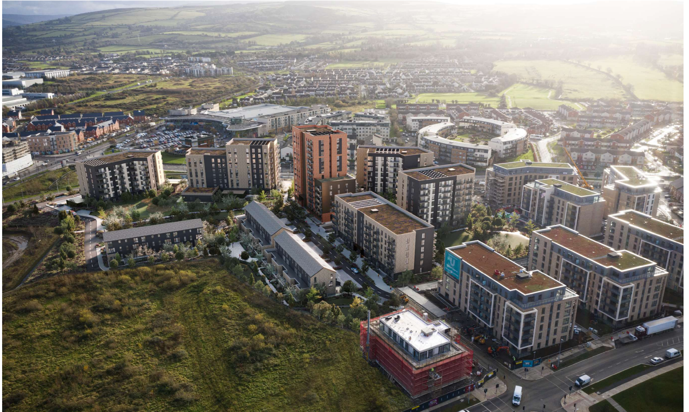
Figure 20 - Aerial view of new Cooldown Commons Quarter
