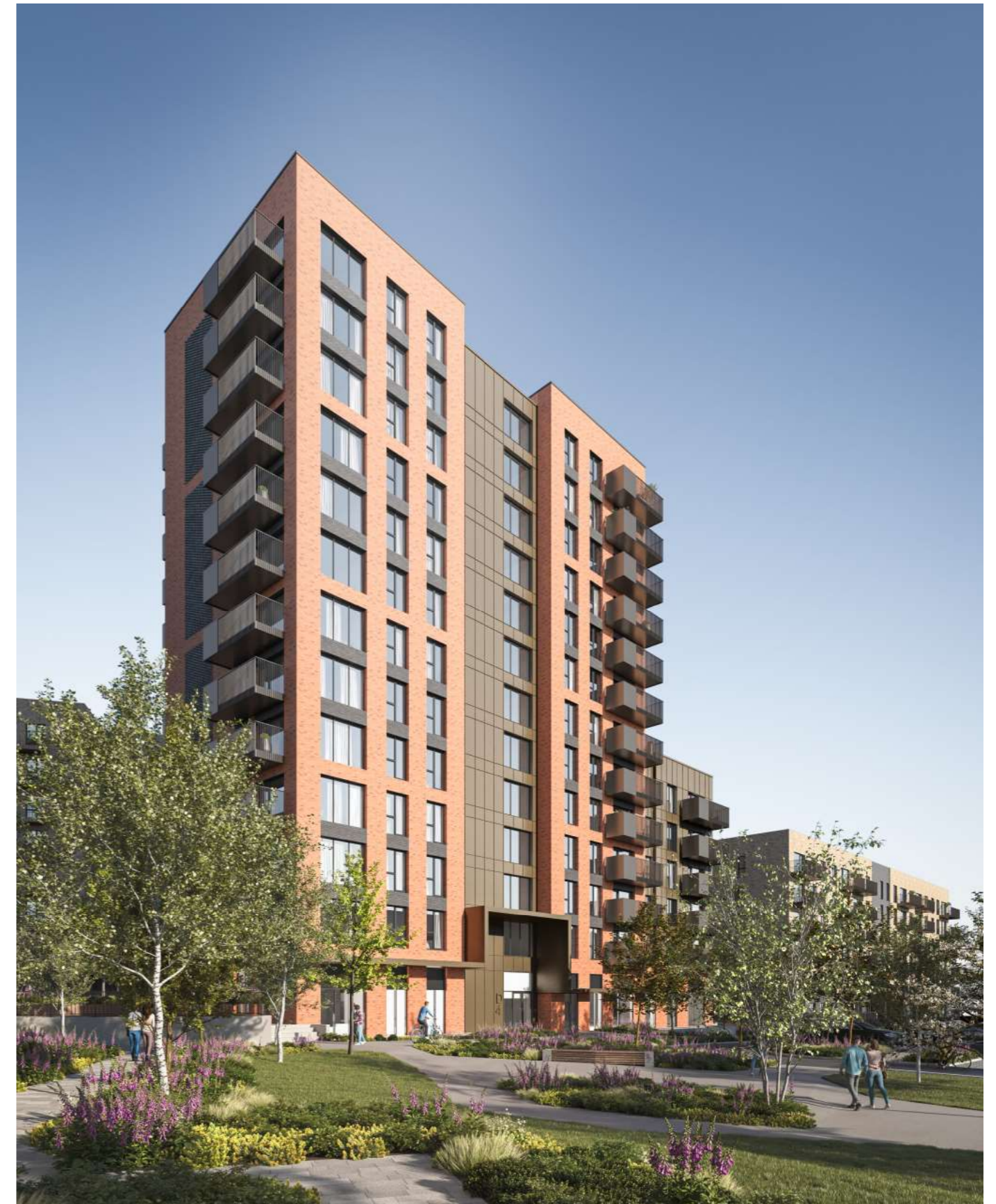
Figure 2 - Close up of Block D4
