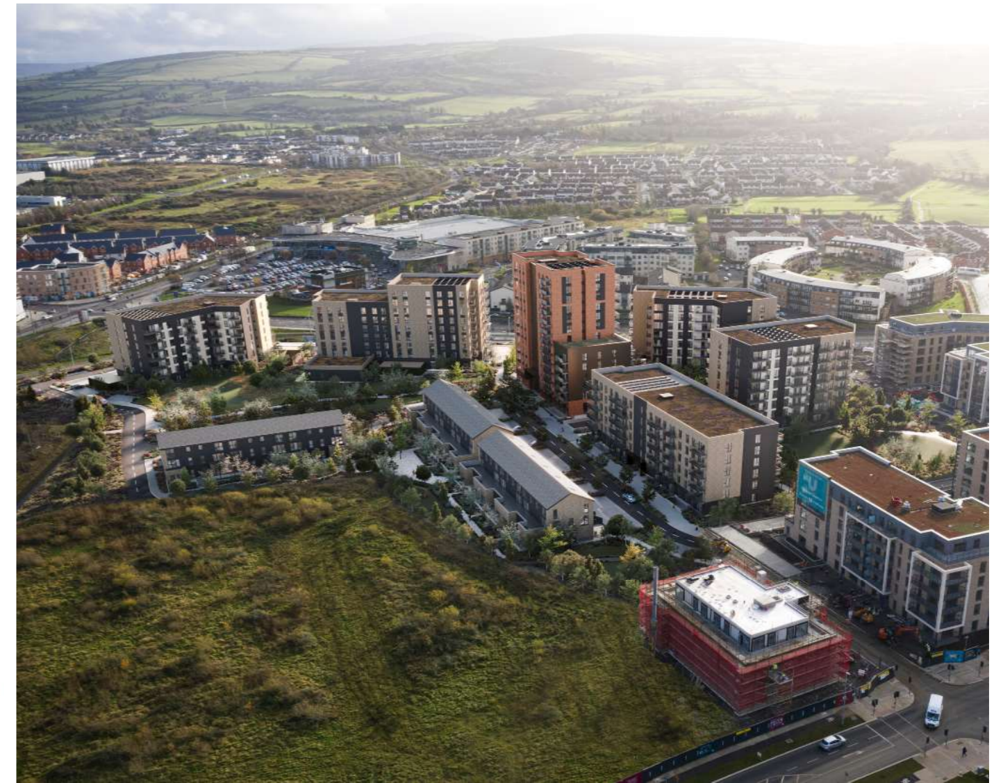
Figure 5 - Aerial view of Cooldown Commons Phase 3
